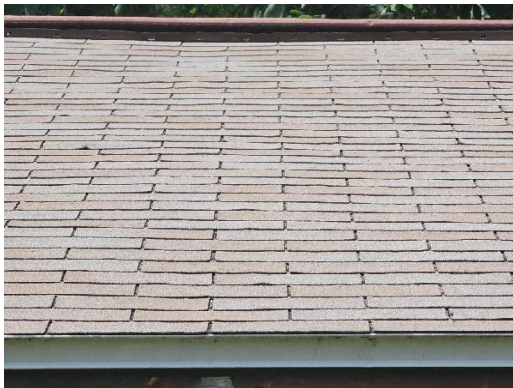
1501-5 Asphalt Shingle/Tar Typical Exterior Roof
