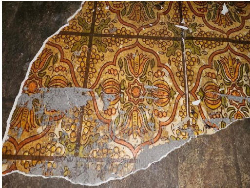
1501-3 Rolled Flooring/Orange (15% Chrysotile) Interior Kitchen (Appx 135 sq ft) Bottom Layer
