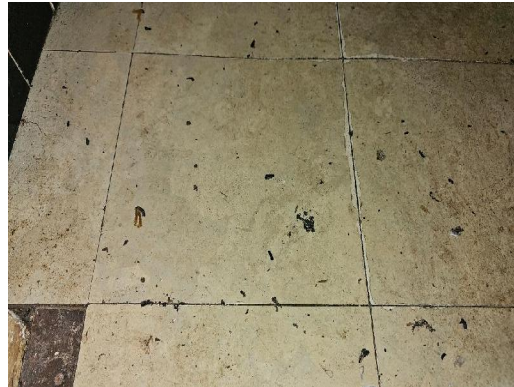
1501-4 12"x12" Floor Tile/Adhesive Interior Bathroom
