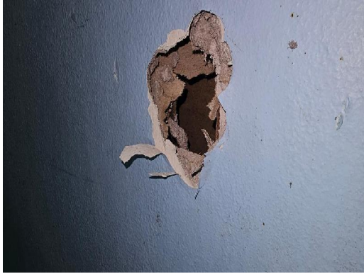
1501-1 Drywall/Joint Compound Typical Interior Walls/Ceilings
